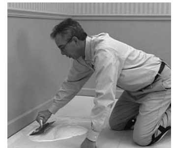
Fig. 4. Apply adhesive and install product.
