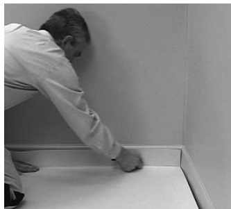
Fig. 2. Cut leaving 1/8" to 1/4" space at perimeter.
